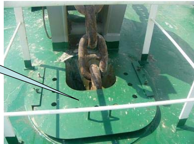
Hawse pipe cover
